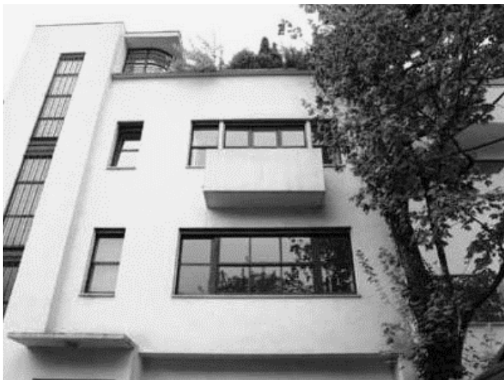
Fig.2.8. Hotel Collinet (1925-1926) Boulogne-Billancourt – Robert Mallet Stevens (1886-1945) © Centre Pompidou
