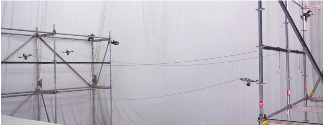
Fig.74 - Processo de Montagem, Aerial Construction, Federico Augugliaro, Prof. Raffaello D'Andrea, 2012. (idsc.ethz.ch, 2017, 9)
