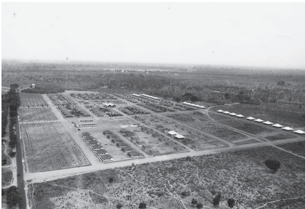
FIGURE 3. The construction of the Ajuda neighborhood, aerial view (1965–1966). Photo courtesy of Prof. Sandra Mula.
